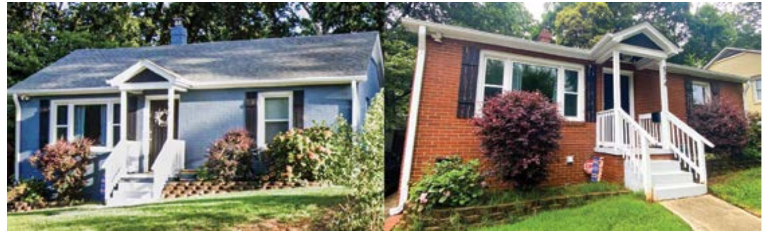
Kingston Avenue – before and after paint removal.
