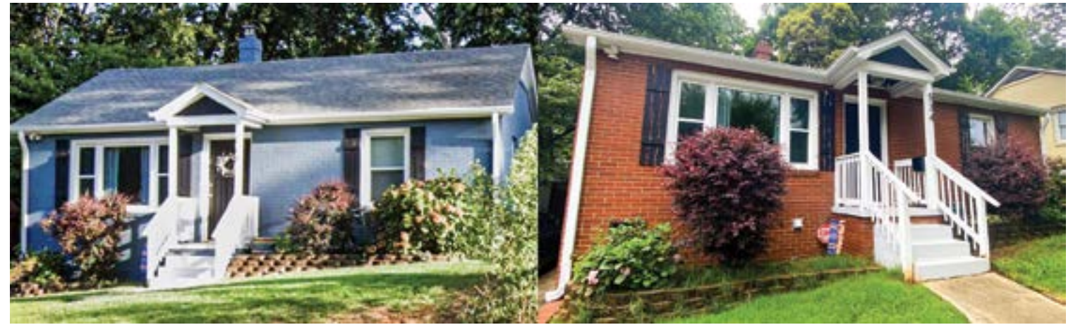
Kingston Avenue – before and after paint removal.
