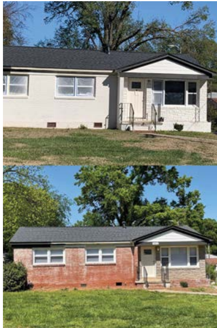
Waddell Street – before and after paint removal.
